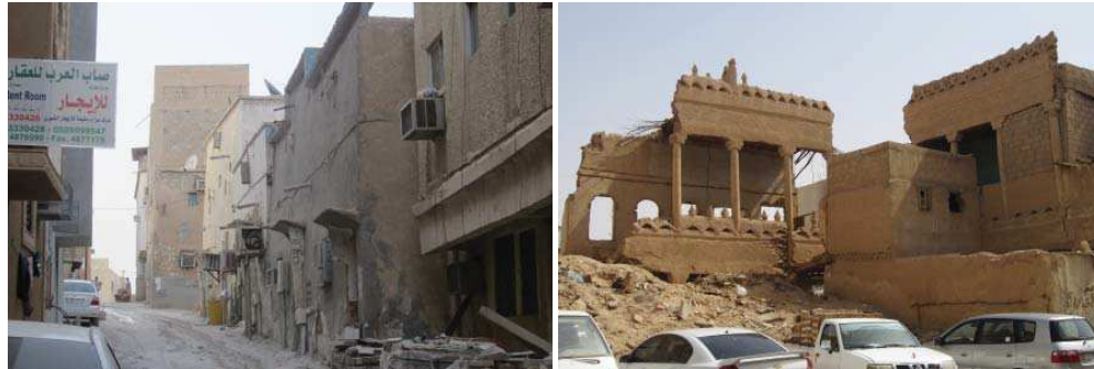
Fig.4: The physical conditions of the buildings in the center of Riyadh. Source: author.
