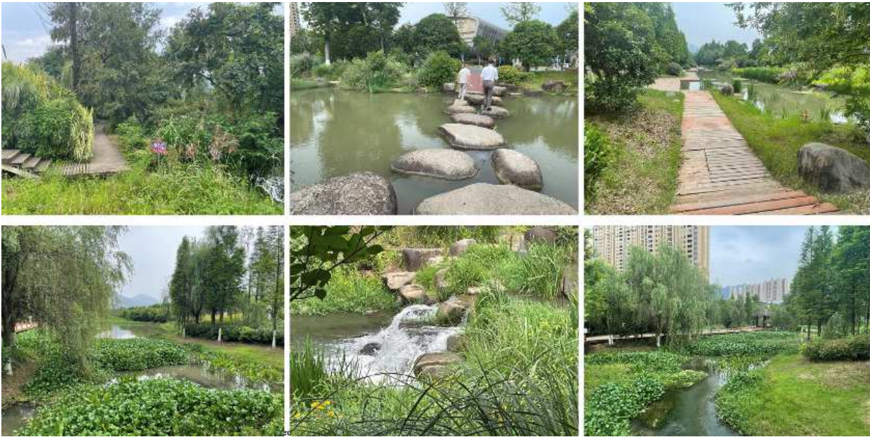
Flood risk reduction. Restored riverside wetlands and green water edges along gentle slopes along the river reduces the risk of flooding. At the same time, they provide a habitat for a diversity of plant and animal species and serve as an amenity for residents during non-flood times. (Photos: Stefan Rau) Source: Asian Development Bank.
