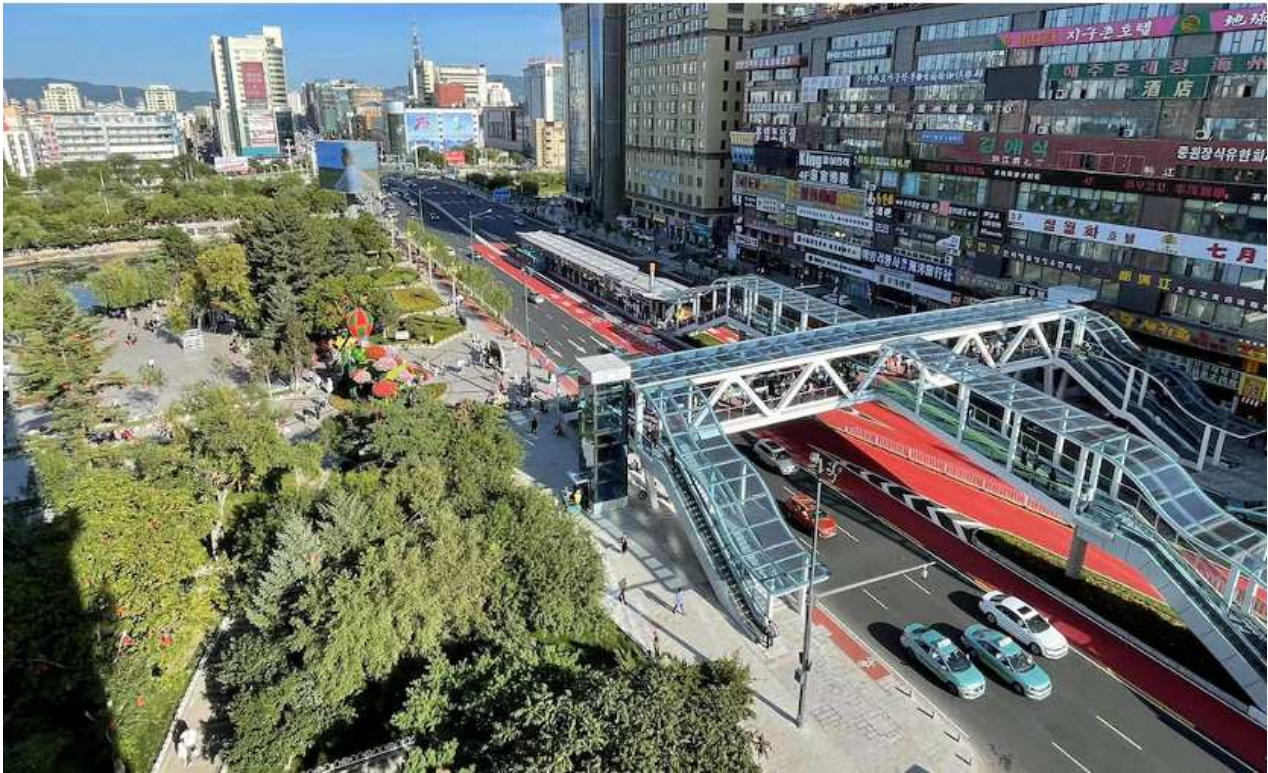
Implemented first phase of the bus-rapid transit with bike paths and sponge city tree planting and road median landscape linking to green parks. Source: Yanji City Government
